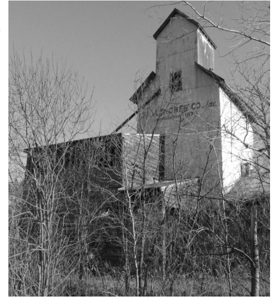
This former I. L. Richer feed plant appears to have been out of use for many years.
