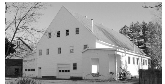
This is the former milk plant as it looks today.
