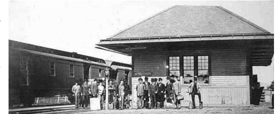
The South New Berlin depot 'back in the day' when it was very much in operation.
