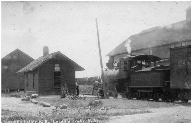
River Forks: station on the left, coal and feed buildings behind it, milk plant on the right behind the train.
