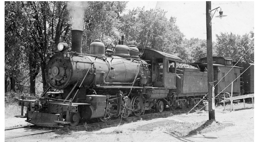
#4 out on the main line. Again, note the wooden frame built into the tender to expand her coal carrying capability. Also note the bobber caboose. The UV had purchased two of these cabooses from the O&W in 1924, and they served the line until replaced in the Forties.
