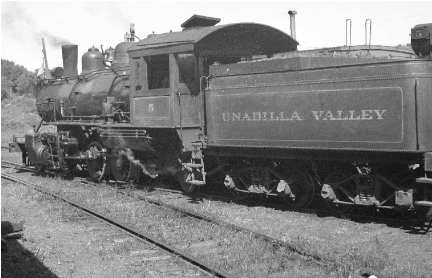
#5 passes the UV station in New Berlin. Not intended as a main line engine, the tenders of the "Prairie" locomotives did not hold much coal, which gave them a fairly short range between coal refills. The wood frame was an effort by the local shop to spare the crew the embarrassment of running out of coal out on the line.
