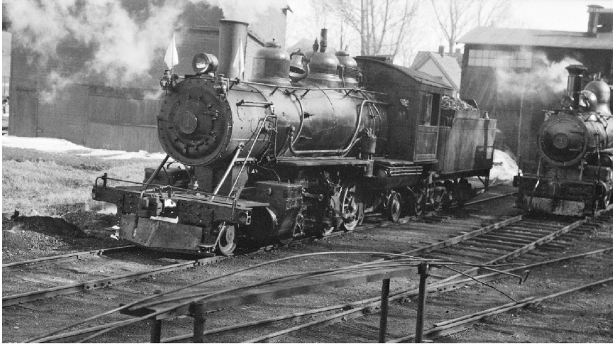
#4 in the UV yard on a cold winter's morning. At her side is Pendragon, both simmering while awaiting the day's activities. In the foreground on the track are several tools used to pull the cinders and ash out of the firebox. Note the wooden framework built into the tender to increase its capacity
