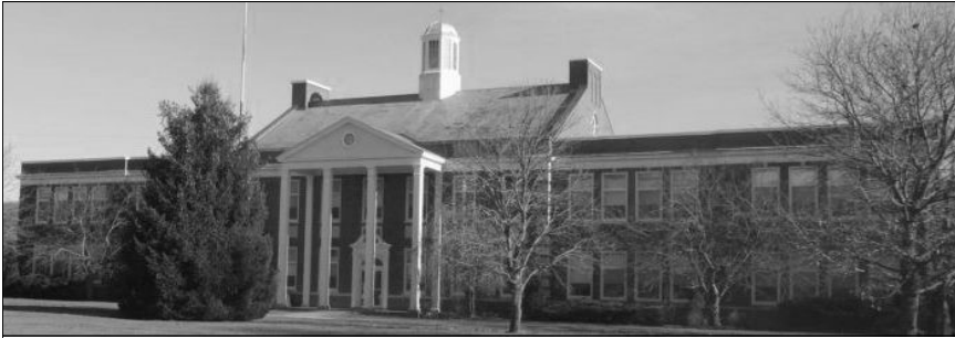
The former South New Berlin Central School (now privately owned).
