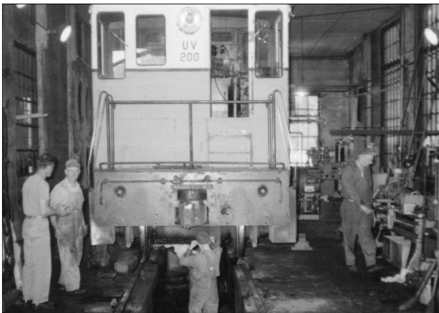
The Shop area of the enginehouse in New Berlin.
