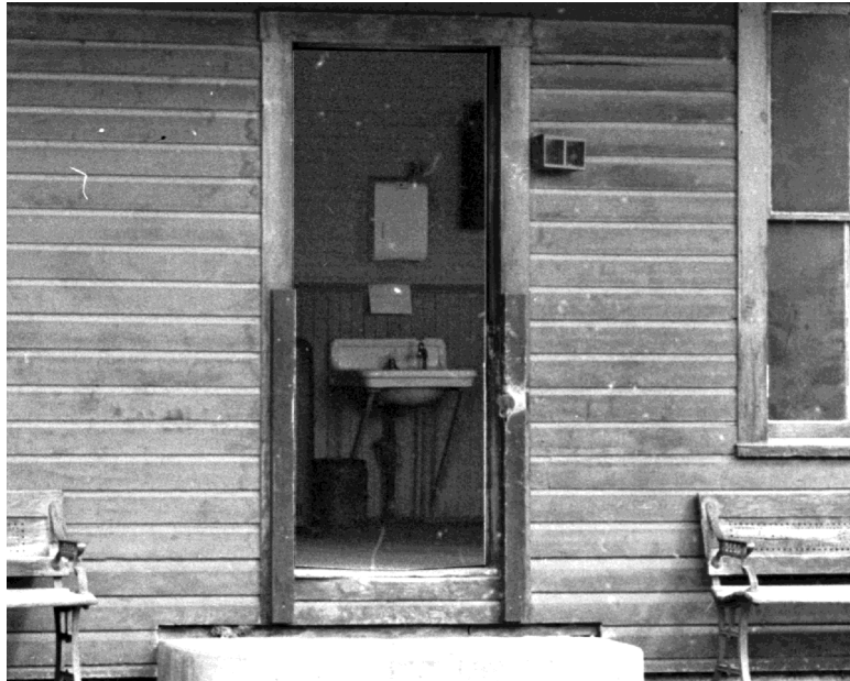
While we know of no pictures of the interior of the depot, this enhanced picture looking in the door gives us an idea of the general appearance of the interior. The passenger depot had vertical wood paneling up to a height of roughly 4', with the upper walls being horizontal boards. Note that the passenger depot floor was not at ground level, but elevated about 18" above ground level, with two steps up to floor level.
