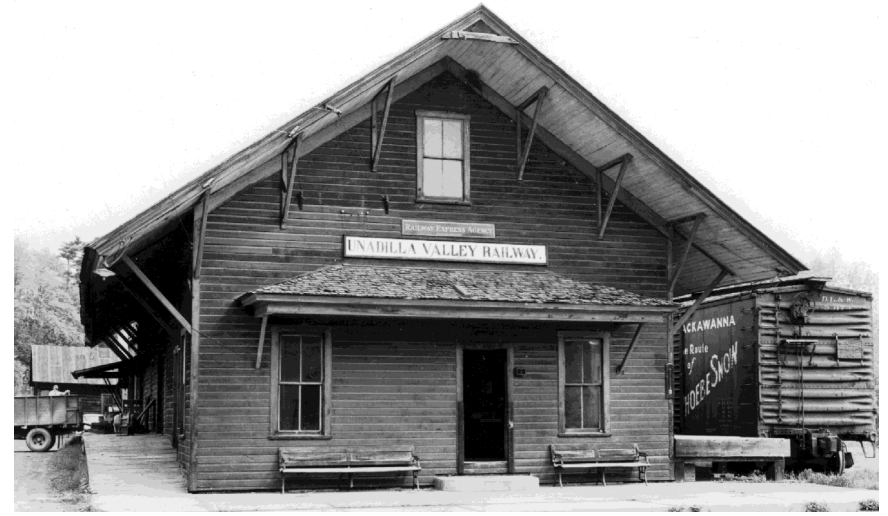
The depot in the Fifties. Note the boxcar being loaded or unloaded on the right, and the truck on the left, taking delivery of feed for a local Purina merchant. The colors of the depot are dark red siding with dark green trim and details. The underside of the roof is either white or light blue.
