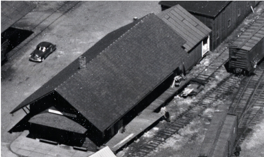
A close-up from the previous picture, showing the overall layout of the depot and the track side loading dock.. Note how the loading dock was built out to facilitate loading and unloading rail cars.
