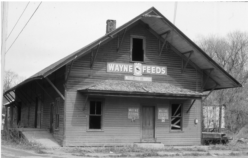
After the UV was abandoned, the depot building was repurposed. Here it is pictured in later years, presumably after Wayne Feeds either went out of business or relocated elsewhere.
